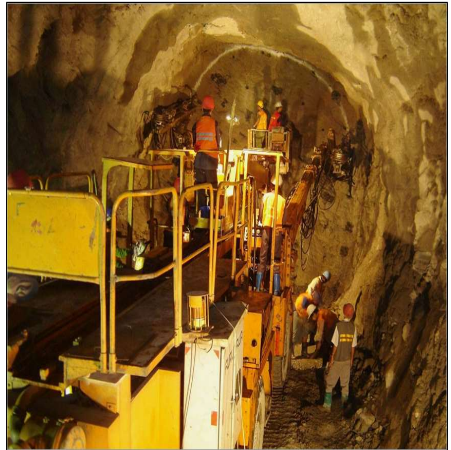
(8) Drilling and blasting
