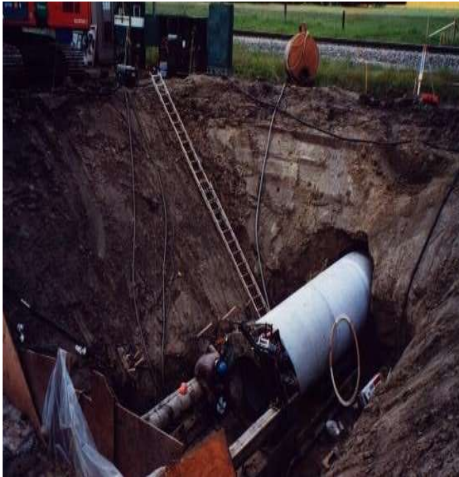
(5) Pipe jacking method
